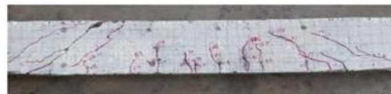
Fig -9: Crack pattern for optimum
