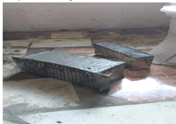
Fig.11: Concreting the Mould
