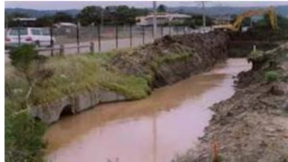
Fig 1: Source of turbid water
