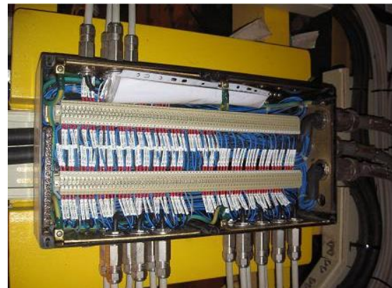
Figure 5. Sample picture of Junction box with field wirings
