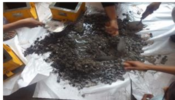
Figure 3. Preparation of concrete mix
