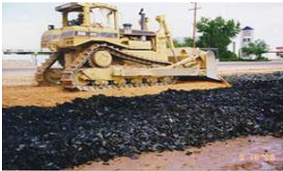
Fig.3. Road embankment constructed with shredded tyres in El Paso, Texas.
