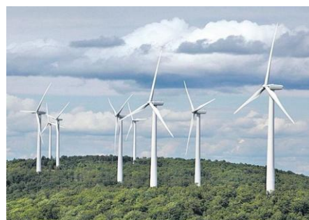
Fig 1.11 Wind Turbines in ANDHRA PRADESH, INDIA
