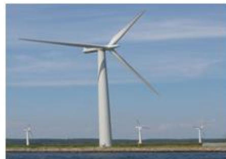
Fig 2.5.7 Three blades HAWT
