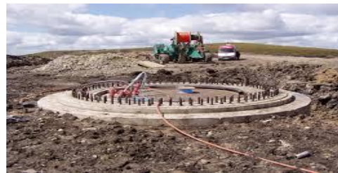
Fig 2.5.4 Foundation for tower
