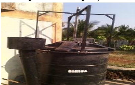
Fig.2 1000 liter Digester setup
