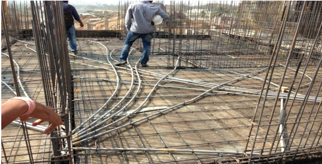
FIG : Horizontal reinforcement of shear wall SHEAR WALL DESIGN USING STAAD PRO: FC : 25.00MPA FY : 415 MPA CONCRETE COVER :25MM MINIMUM REIN FORCEMENT RATIO
