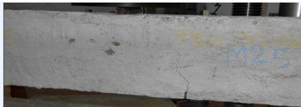
Fig: 4.16: M25-Large beam before Loading & after loading
