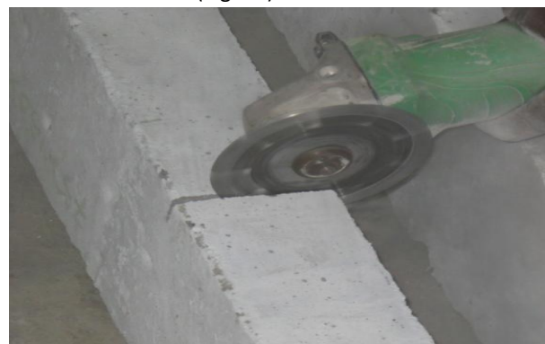
Fig 2.1: cutting a beam with marble cutter
