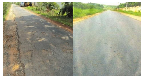
Fig.2. Comparison of Plastic Road with Conventional Road
