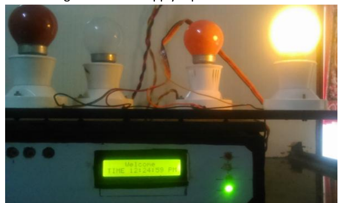
Fig 9: Electrical supply is provided to area 1 on 12:24PM
