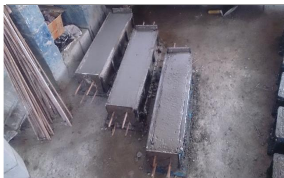
Fig. 2 Casted specimen of beams with reinforcement
