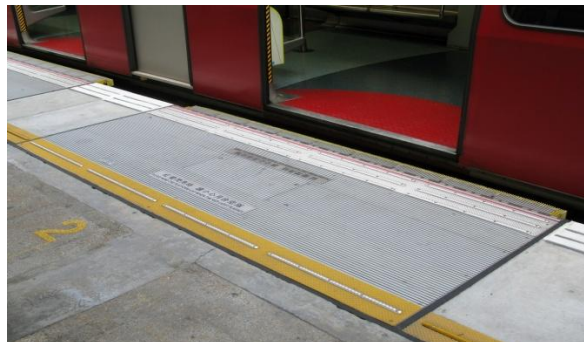
Fig 5: MTR Lo Wu Station Platform Gap Fillers (Hong Kong) which extend slightly over the platform edge and reduce the gap
